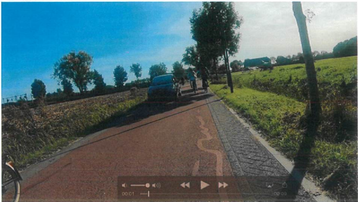
Figure 8 Example of optical narrowing of the road. The different colour bricks encourage everyone into the middle of the road, which tends to slow all traffic down.
